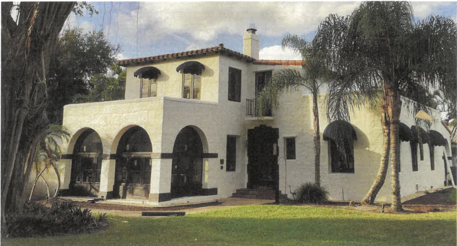
One of the first in Mizner’s doomed Boca Raton development, this Mediterranean-inspired house, designed for film executive Fred Aiken, is now historically designated.
